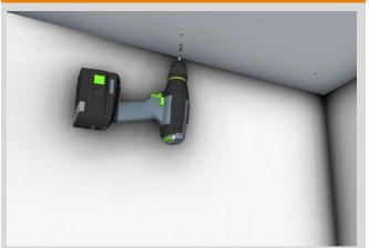
Drill holes at the marked points and insert the dowels.
