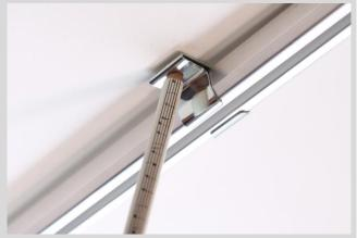
Position the rail as required and mark the drill holes through the hole in the ceiling bracket.
