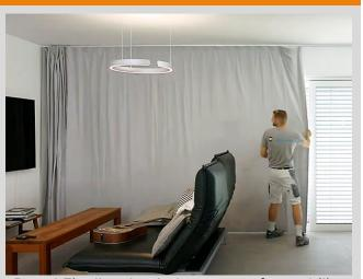
Done! Finally, check the system for stability and good roller running properties.
